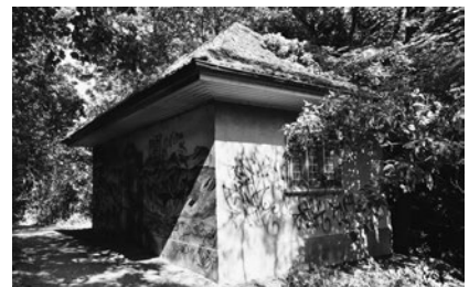
13. Reservoir Malvaux, Leubringen
