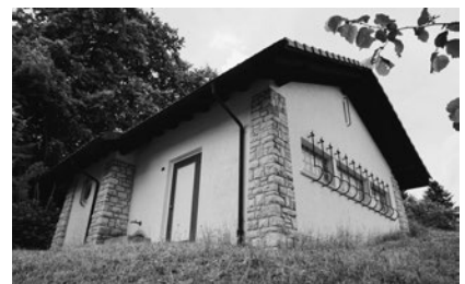
18. Pumpstation, Belairweg 16, Magglingen
