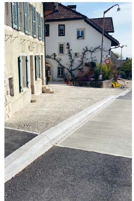
Pflastersteine Route Principale 42/44
